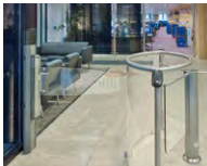
07 ENTRY AND EXIT SYSTEMS
